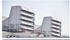
combined-cycle facilities where the steam is raised through using the exhaust heat from the gas-fired combustion turbines.
